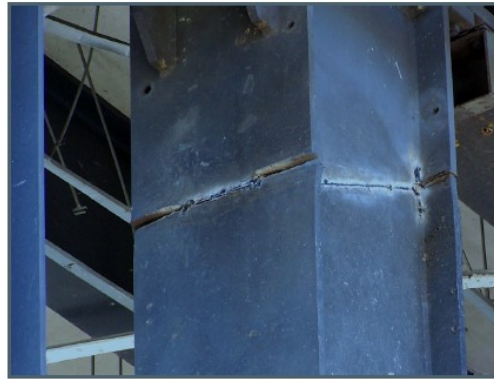
Fig.3 Cut after two Blast attempts
