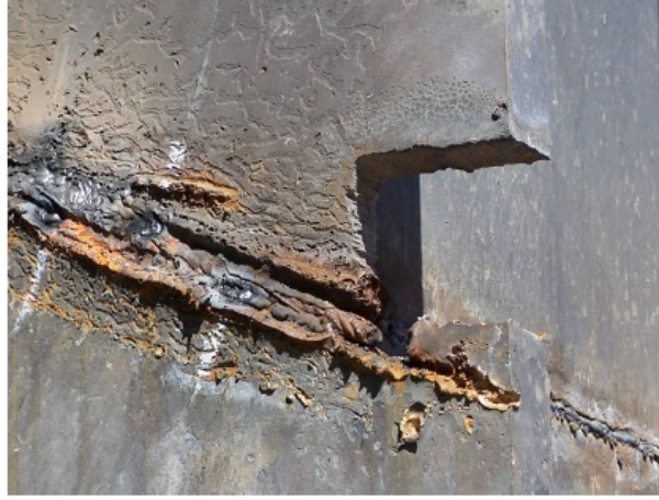
Fig.7 Insufficient Cut After Blast Attempt
