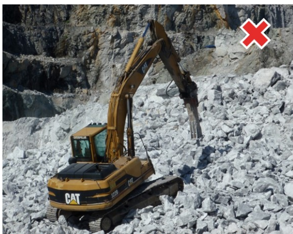
Figure 1: wrong and unsafe oversize hammering treatment.
