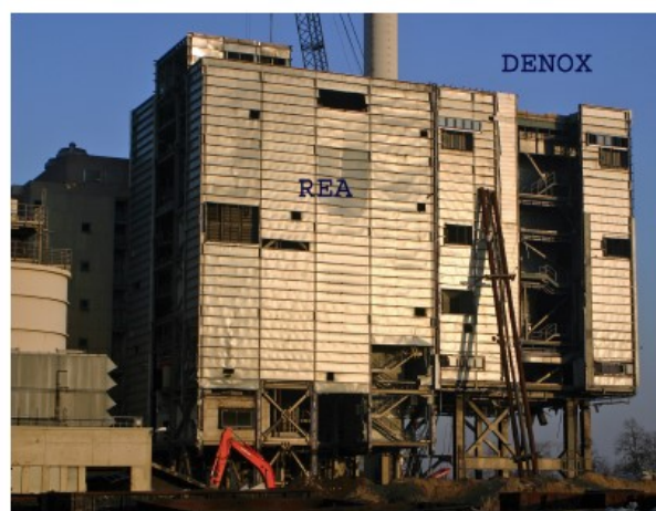
Fig.2 Power Station View Two
