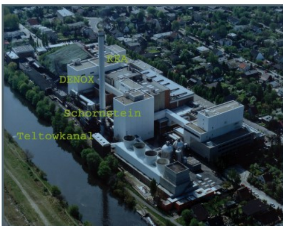
Fig.1 Power Station-View One
