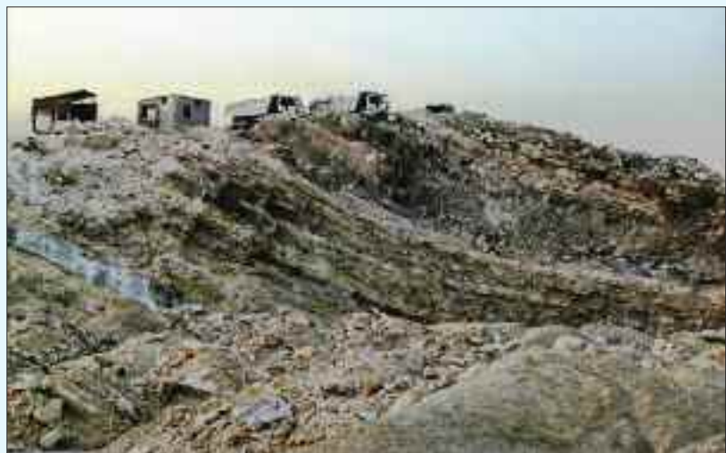
Figure 3. High wall showing structural discontinuities at Dhofa- Mining gypsum quarry in Raweya.
